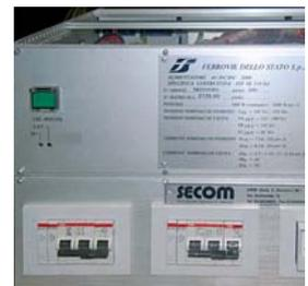
For the substation SECOM developed natural air cooled power rectifier at 3000 Vcc to fed the eletrical line network while special protection devices are installed along the railway tracks to avoid sudden and dangerous overvoltages SECOM also developed switching power supplies with high
